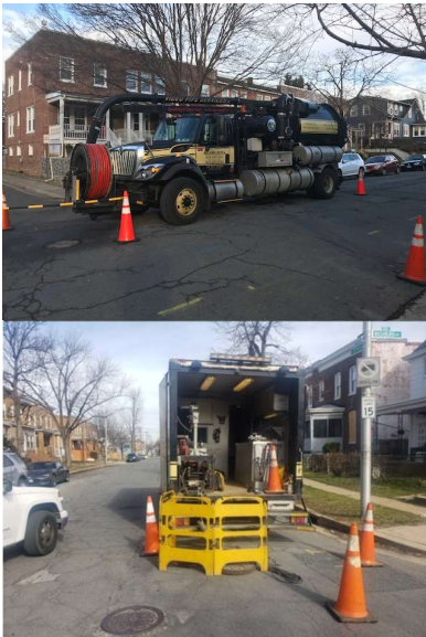
Example of typical CCTV inspection truck setup. In order to conduct CCTV inspections two trucks are needed, one at either end of the sewer.
